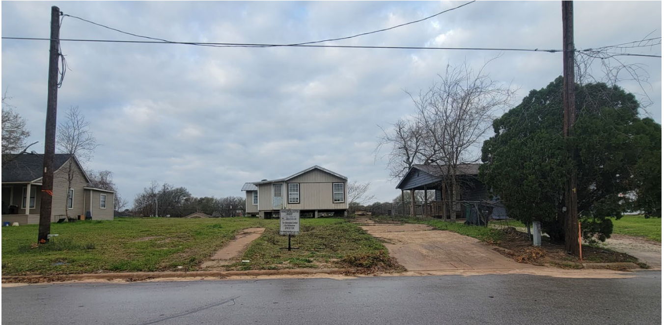
Subject property – the electric poles are at the property lines
